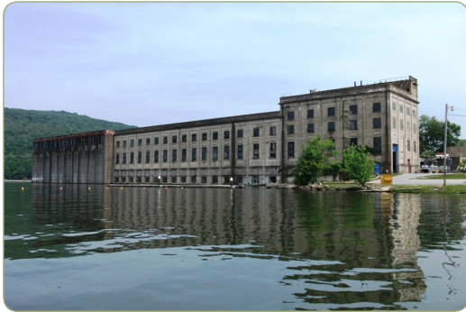
Surviving powerhouses from Hales Bar Dam.
