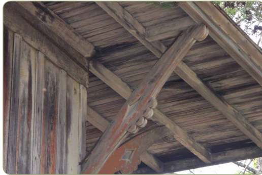
Detail of bracket supporting roof.
