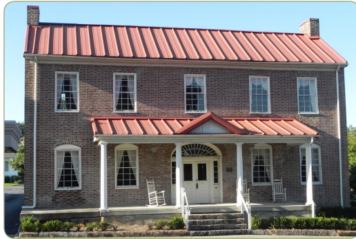
Historic John Bridgman House on Spring Street, ca. 1810s, listed in the National Register of Historic Places.
