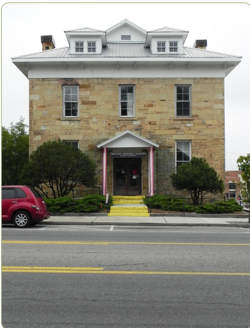
The old Cumberland County Courthouse on South Main Street houses the Military Memorial Museum of the Upper Cumberland.
