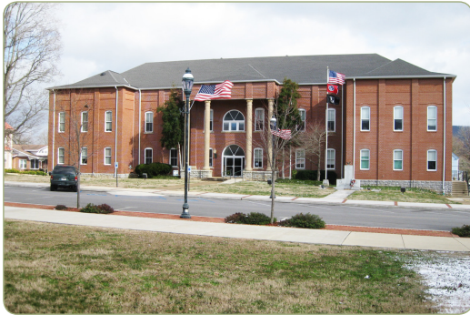
1910 Bledsoe County Courthouse with additions.
