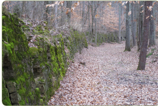
Coke ovens stretch far into the distance.
