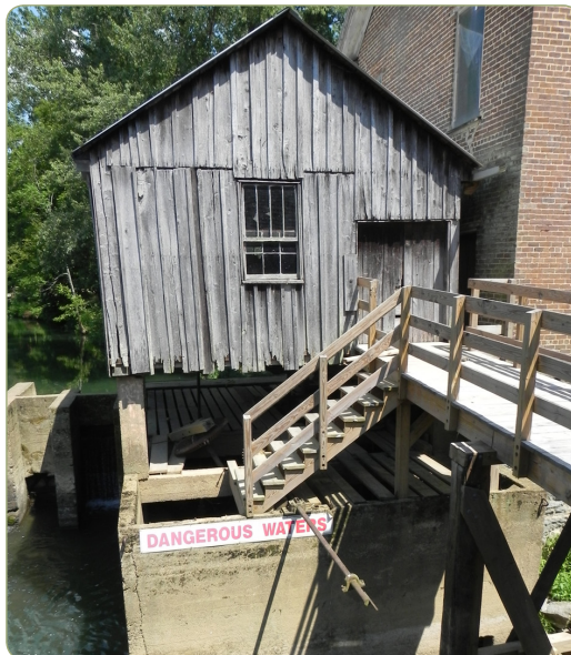
Turbine house at the rear of the mill.
