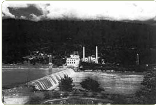
Historic view of Hales Bar Dam.
