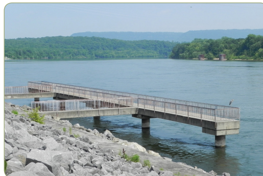
Fishing pier at south bank recreation area.
