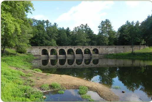
The bridge and dam at Byrd Lake was the largest stone structure constructed by the CCC.
