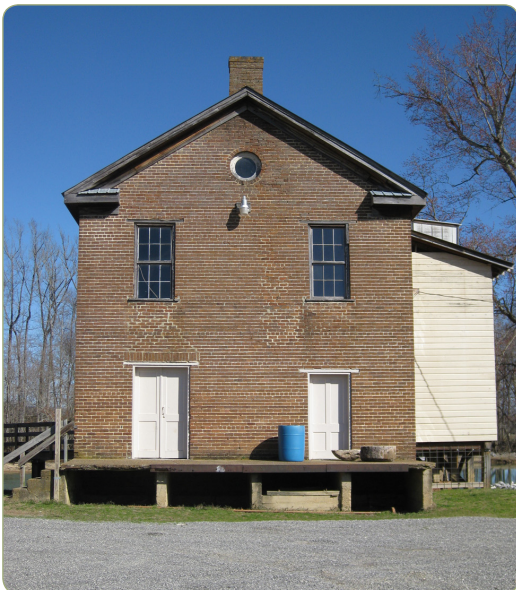
The beautiful brick façade of the historic mill.
