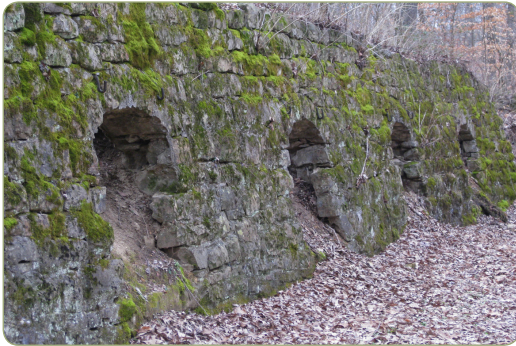
Four of the more than 268 coke ovens constructed at the site.
