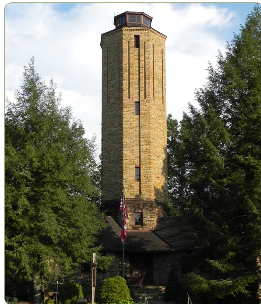
Cumberland Homesteads Tower
